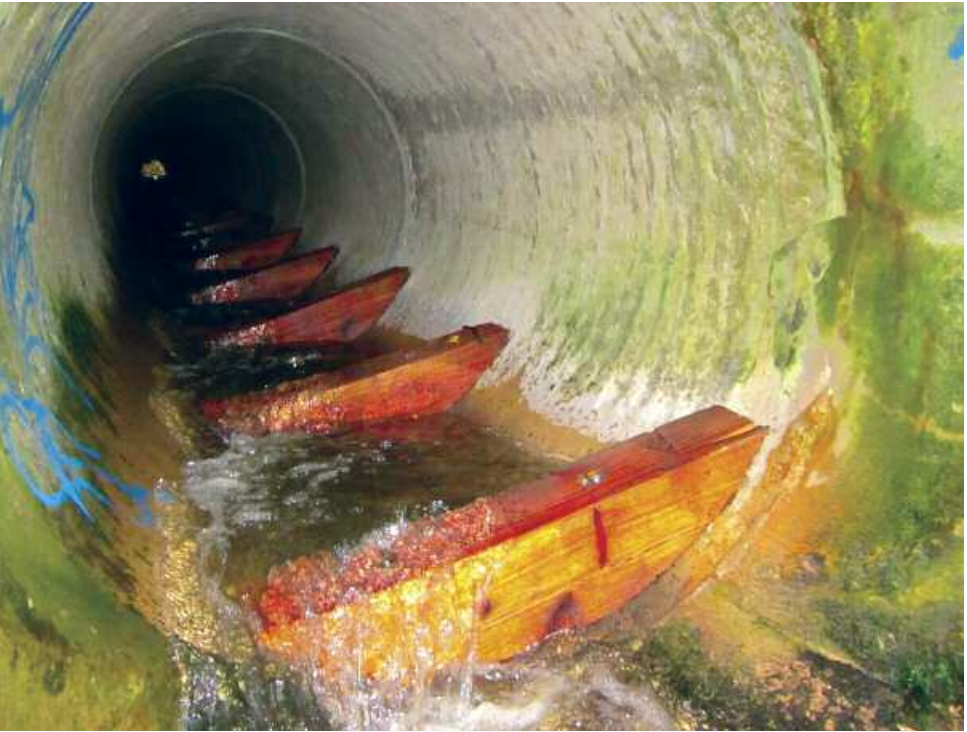
above: Baffles installed in the culvert under NW Marine Drive.
